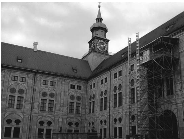
Image 8 Scaffolding in the Emperor’s Court in the Munich Residence
