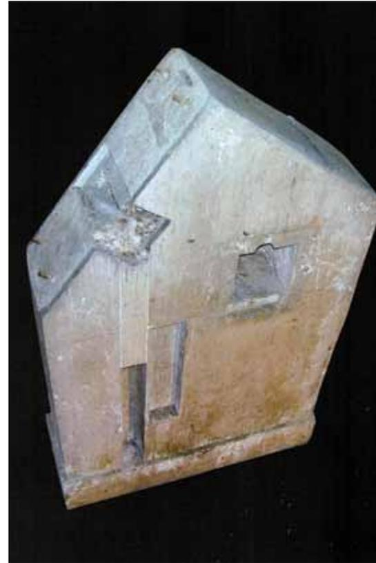
Fig. 3 The cut stone pier of 'Armagh Marble' as it appeared prior to the restoration of the 15-inch telescope showing the recesses for the clock drive in its earlier and later positions and for the weights.
