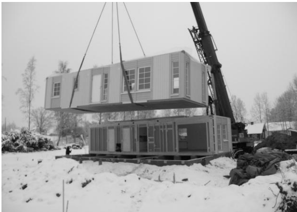
Picture 2: Prefabricated modules for single family house are assembled on-site.
