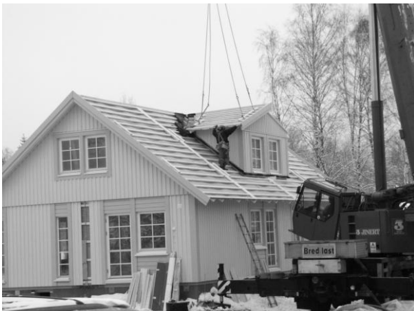
Picture 3: Prefabricated dormer window is assembled on-site.
