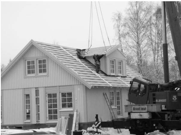
Picture 3: Prefabricated dormer window is assembled on-site.
