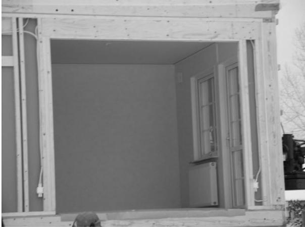
Picture 1: Prefabricated module for single family house with already installed heating and ventilation system and other interior fittings. Arrival on-site.
